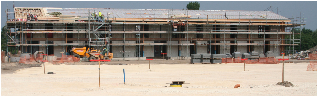
Work on York's Eco-depot October 2006 © Christian Vassie
